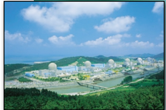
Hanbit Nuclear Power Plant.
