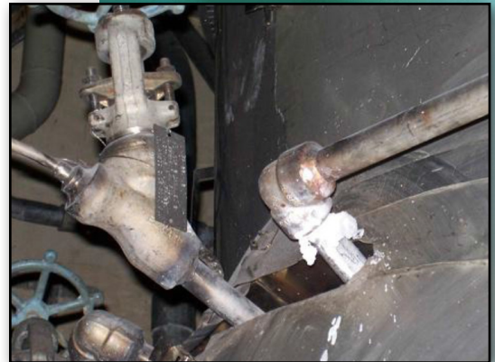
Weld overlay was applied to a socket weld in the reactor coolant system at AEP's DC Cook nuclear plant.
