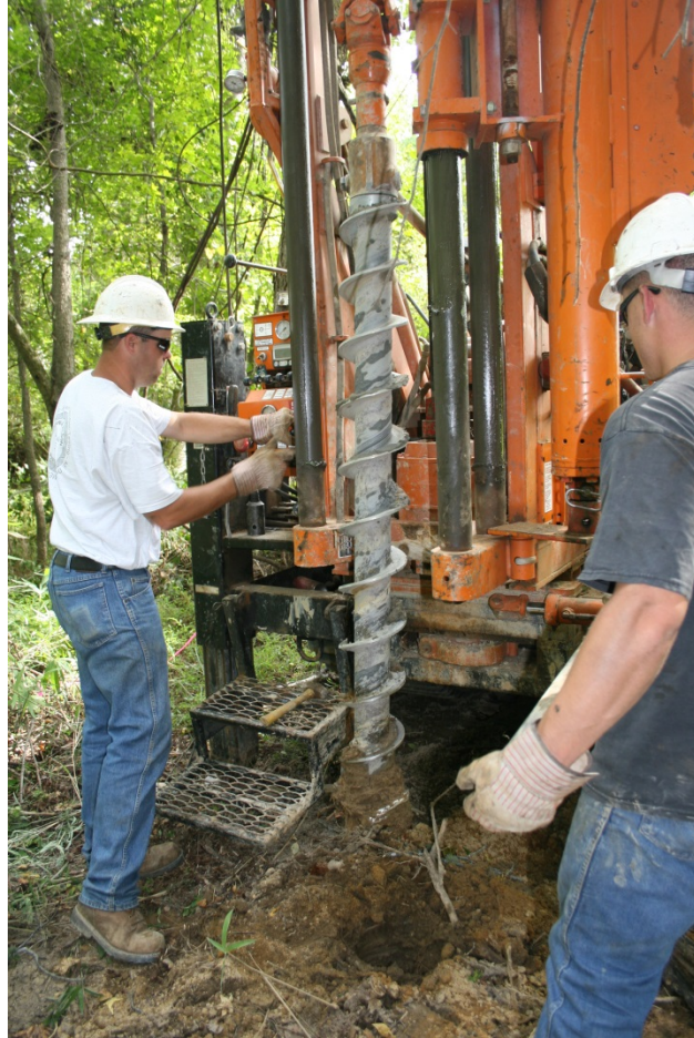
Figure 7-1 Soil testing using a drill rig [54]
