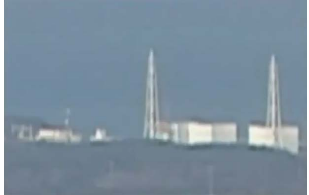
Figure 4-4 1F1 Paneling Blows Off
