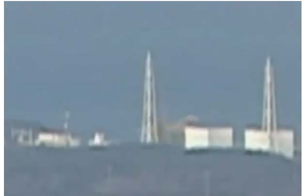
Figure 4-6 1F1 Possible Collapse of Roof
