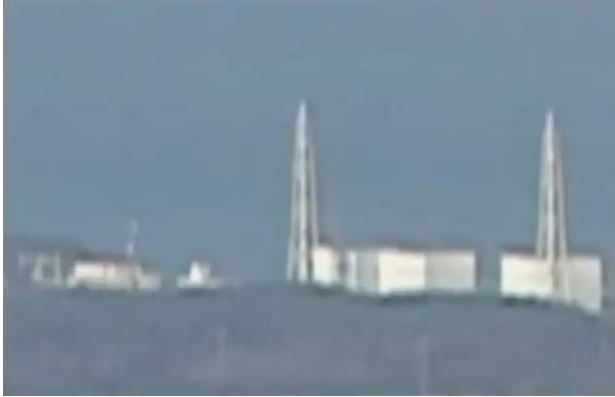
Figure 4-3 1F1 Prior to Explosion
