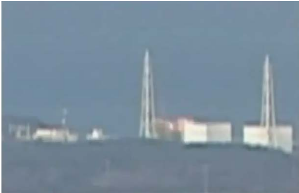
Figure 4-5 1F1 Hydrogen Explosion
