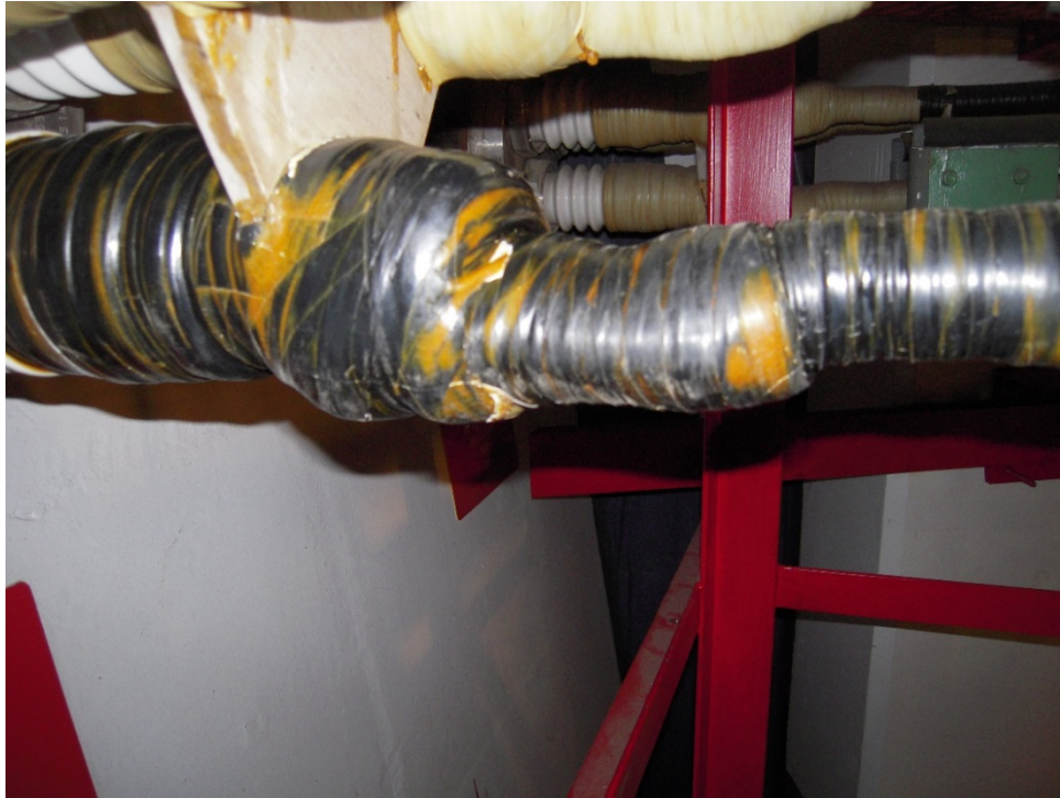
Figure 4-4 Noticeable overheating of the C phase penetration. Note the tan color of the parallel cables in the background.
