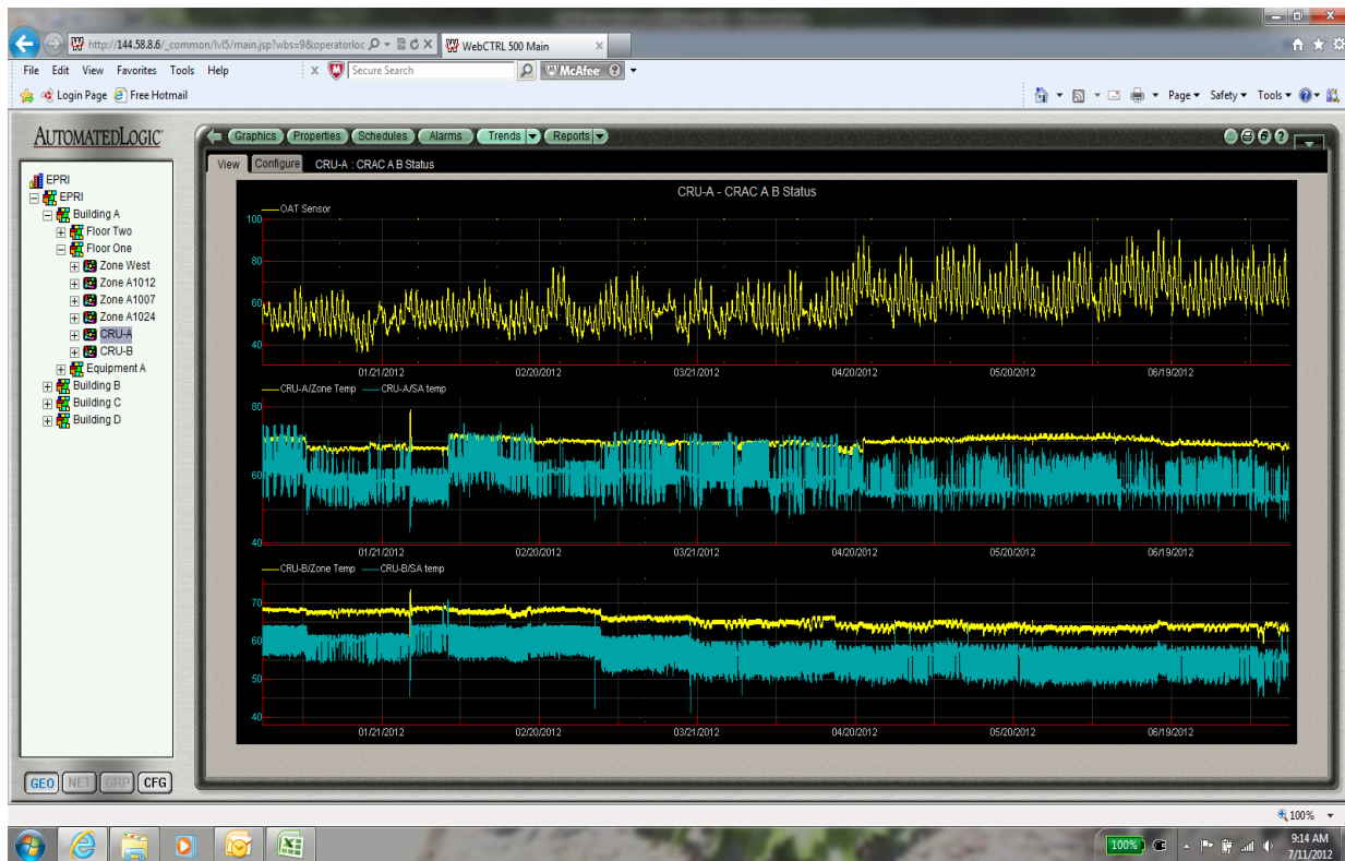
Figure 4-4 Snapshot of the EPRI DX CRAC unit's performance
