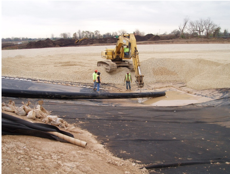
Figure 4-2 Sideslope riser pipe being installed in a leachate collection sump [17]
