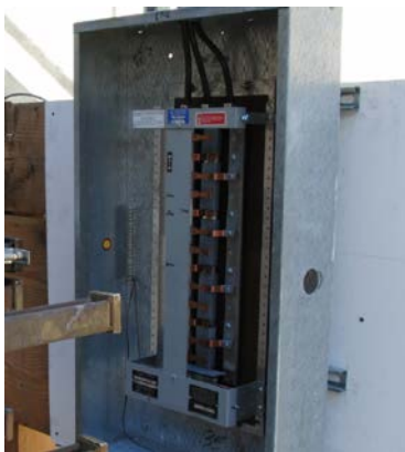
Figure 2-13 Examples of 480-V equipment with borderline arc sustainability
