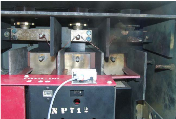
Test ID 43: AΦ-BΦ-CΦ 20AWG with Barrier - 0.34 cycles
