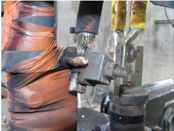
Test ID 56: CΦ-BΦ cable; 1.09 cycles
