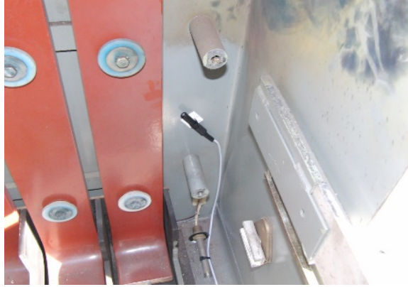
Figure 4-3 Torpedo sensor on the back wall
