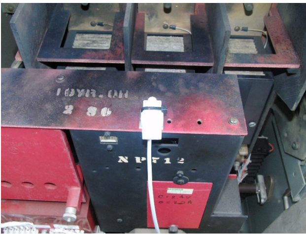
Figure 4-1 Omnidirectional sensor at the top of the breaker module
