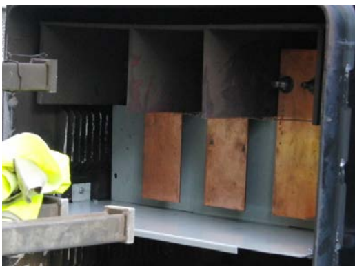
Figure 2-14 Examples of 480-V equipment with sustained arcing
