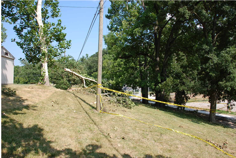
Figure 1-1 Damage to a single phase distribution line caused by impact of a branch from an American sycamore ( Platanus occidentalis ) tree.
