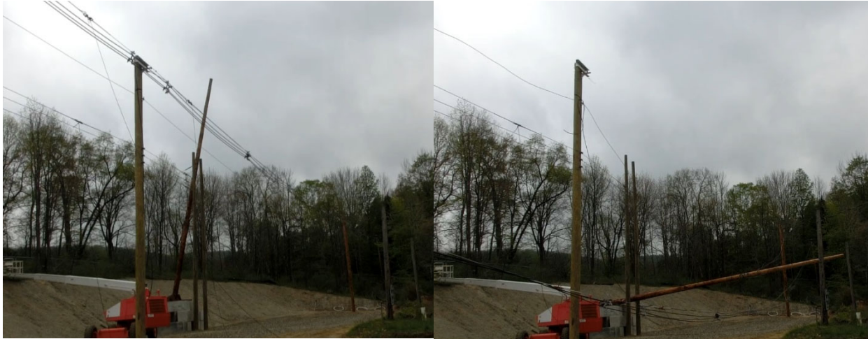
Figure 12-4 Position of spacer cable before and after test
