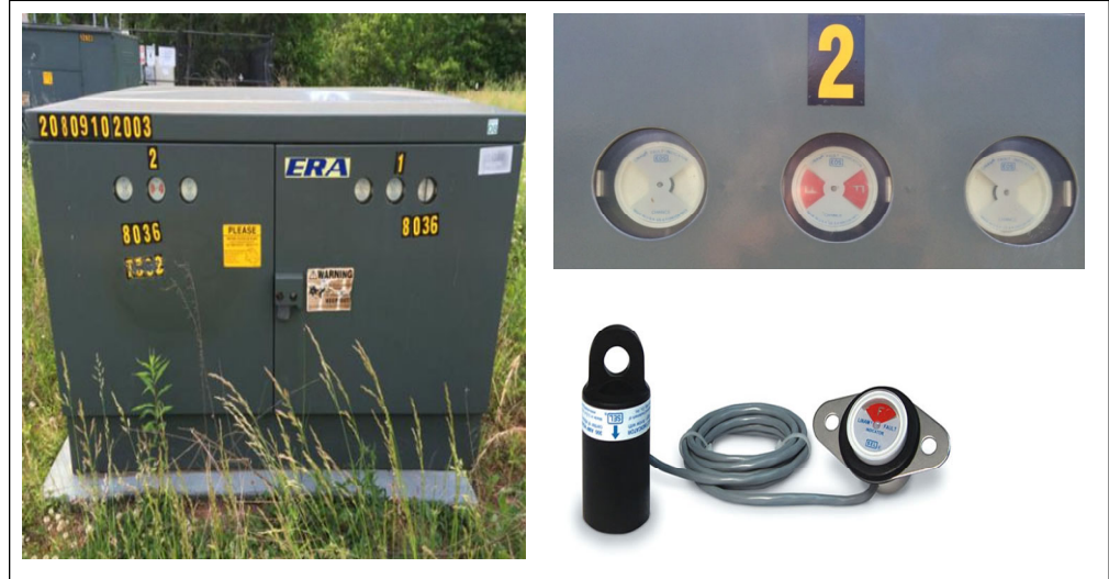
Figure 13-1 Typical Underground Faulted Circuit Indicators [11]
