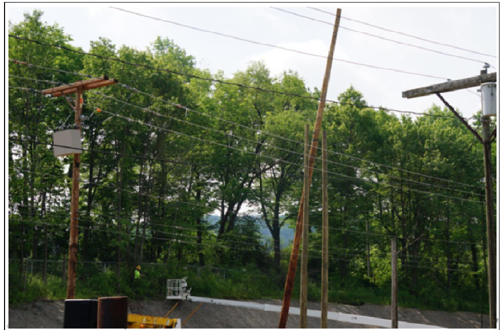
Figure 5-7 Testing of break-away connections to protect DA poles
