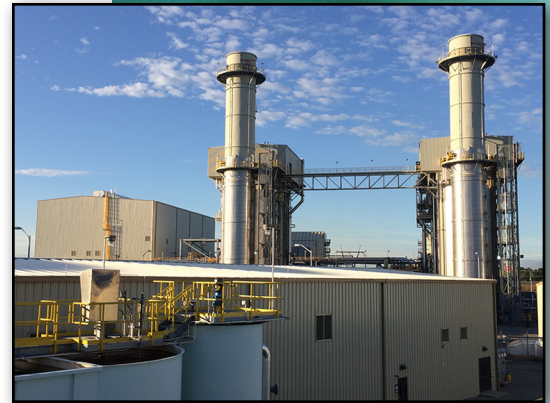
A view of the Cane Run Unit 7 HRSGs and steam turbine building from one of the fast-start clarifiers.
