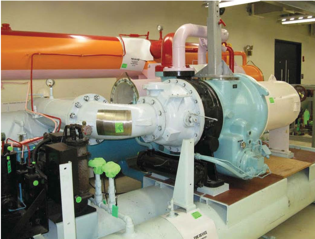
Figure 5-4 Example of Centrifugal Chiller with Hermetically Sealed Motor
