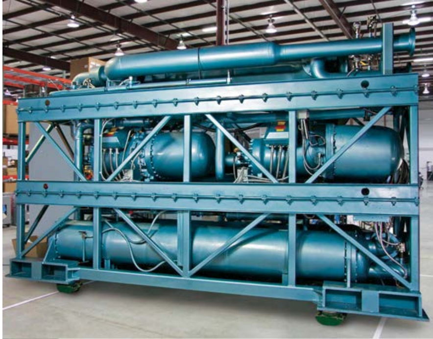
Figure 2-4 A Large Replacement Chiller with Modular Segmented Design
