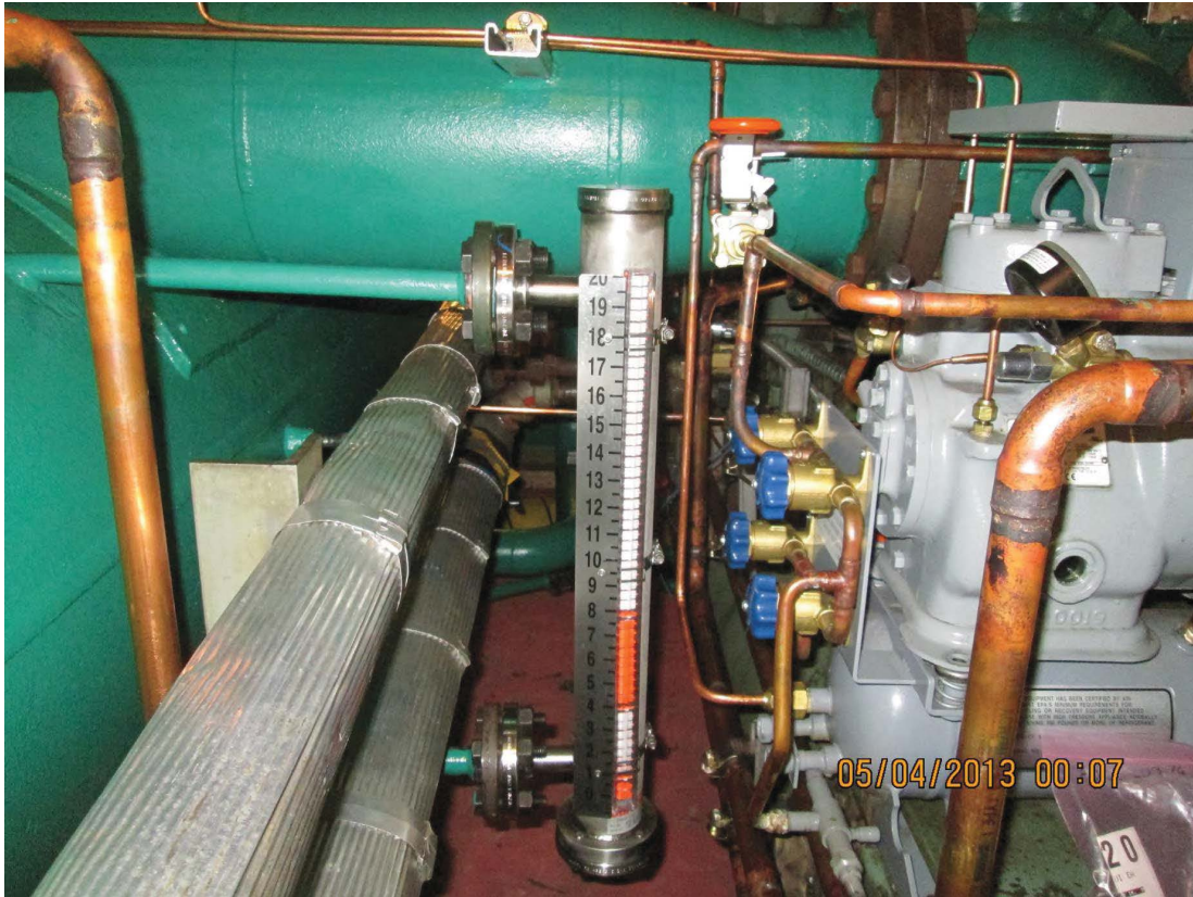
Figure 5-6 Chiller Tubing After Refurbishment
