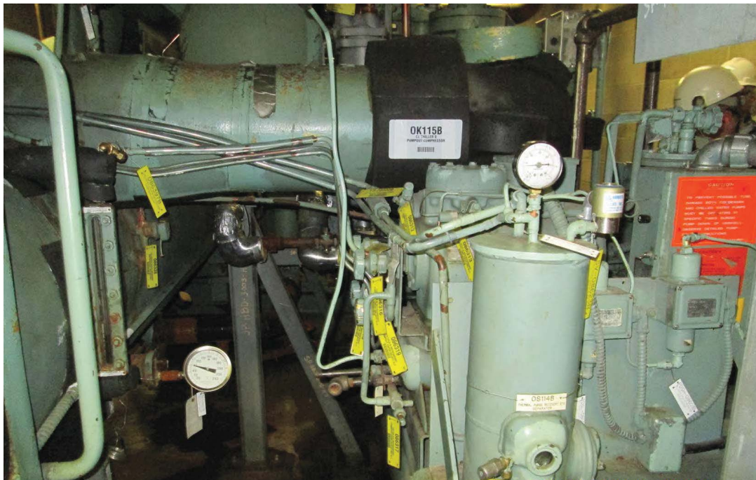
Figure 5-5 Poorly Routed and Supported Chiller Tubing Prior to Refurbishment
