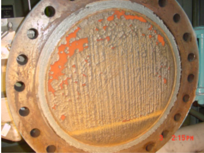
Figure 10-5 Condensate Polisher Resin Trap [6, 27]
