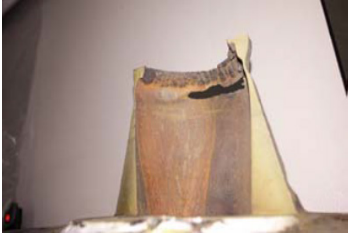
Figure 8-21 Steam Line – Two Phase Flow Accelerated Corrosion [29]
