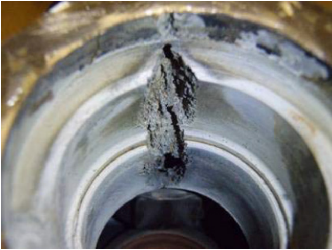
Figure 2-22 Steam Generator Blowdown – Downstream of Throttled Gate Valve – Cavitation Erosion [5]
