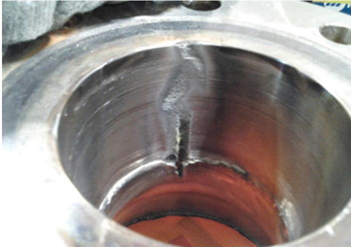
Figure 6-5 Stainless Steel Expander – Steam Cutting Erosion (Photo Courtesy of TVA)
