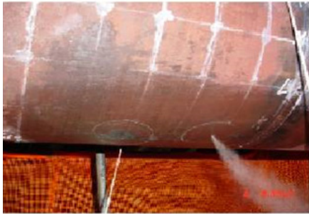
Figure 4-14 Through Wall Leak in Chrome-Moly Extraction Steam Header Diagonally Opposite to MSR Drain Lines [3, 8]
