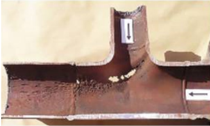
Figure 2-18 Tee and Downstream Pipe – Cavitation Erosion [3, 8]
