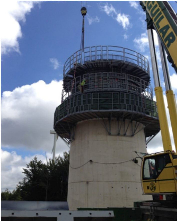
Figure 6 – Climbing formwork elements
