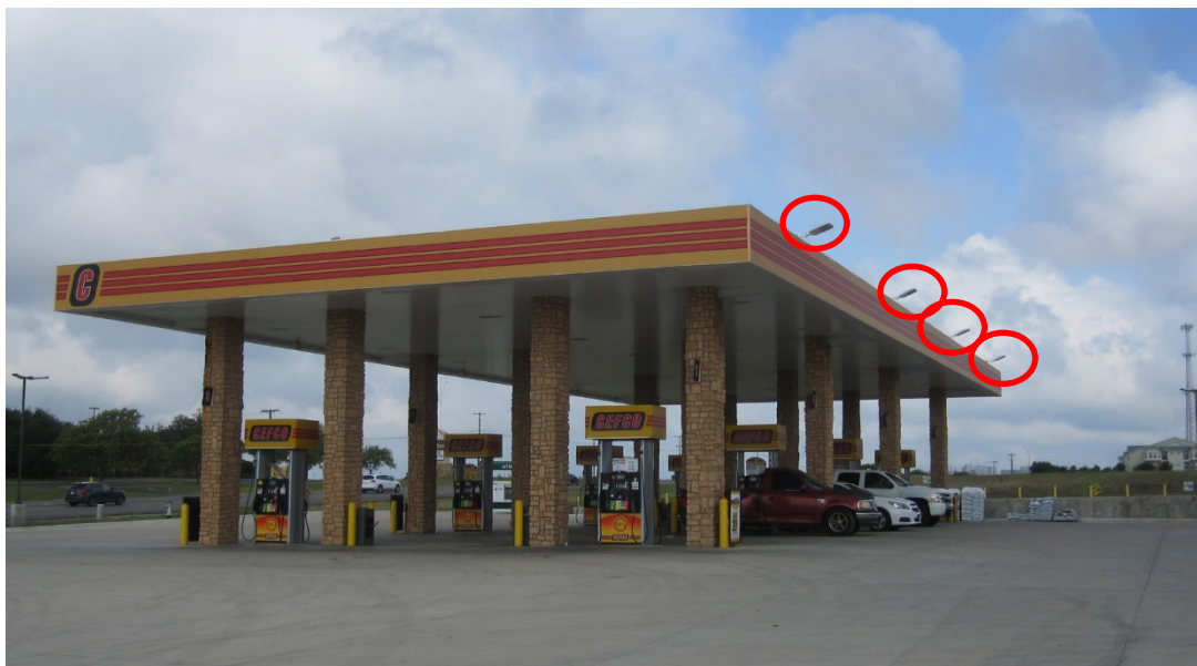
Figure 2-9 Angled LED area lights highlighted in red
