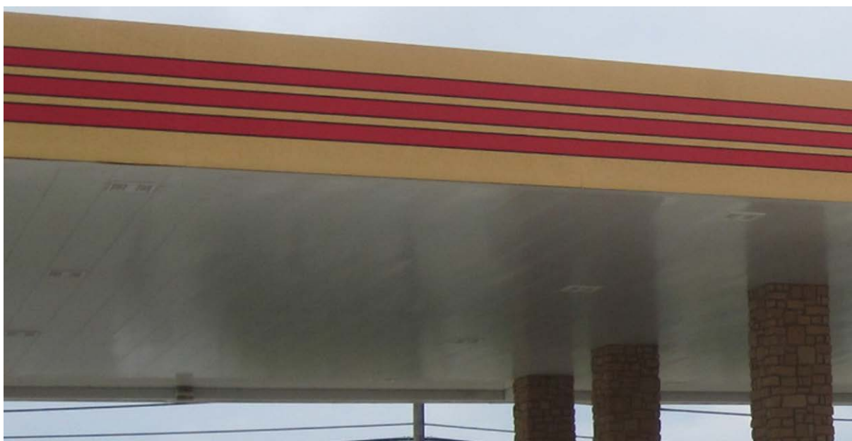
Figure 2-10 Flush-mounted LED canopy lights
