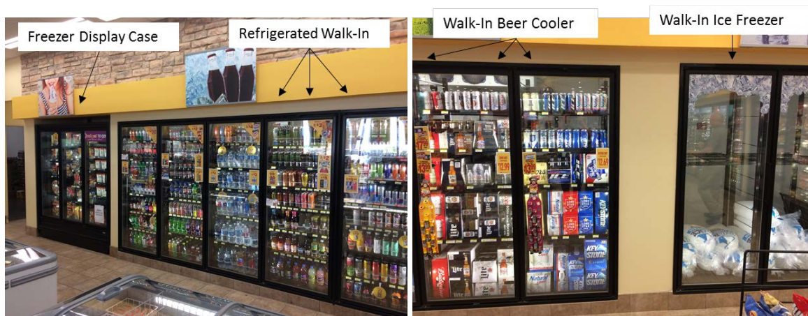
Figure 2-2 Configuration of refrigerated and freezer display cases
