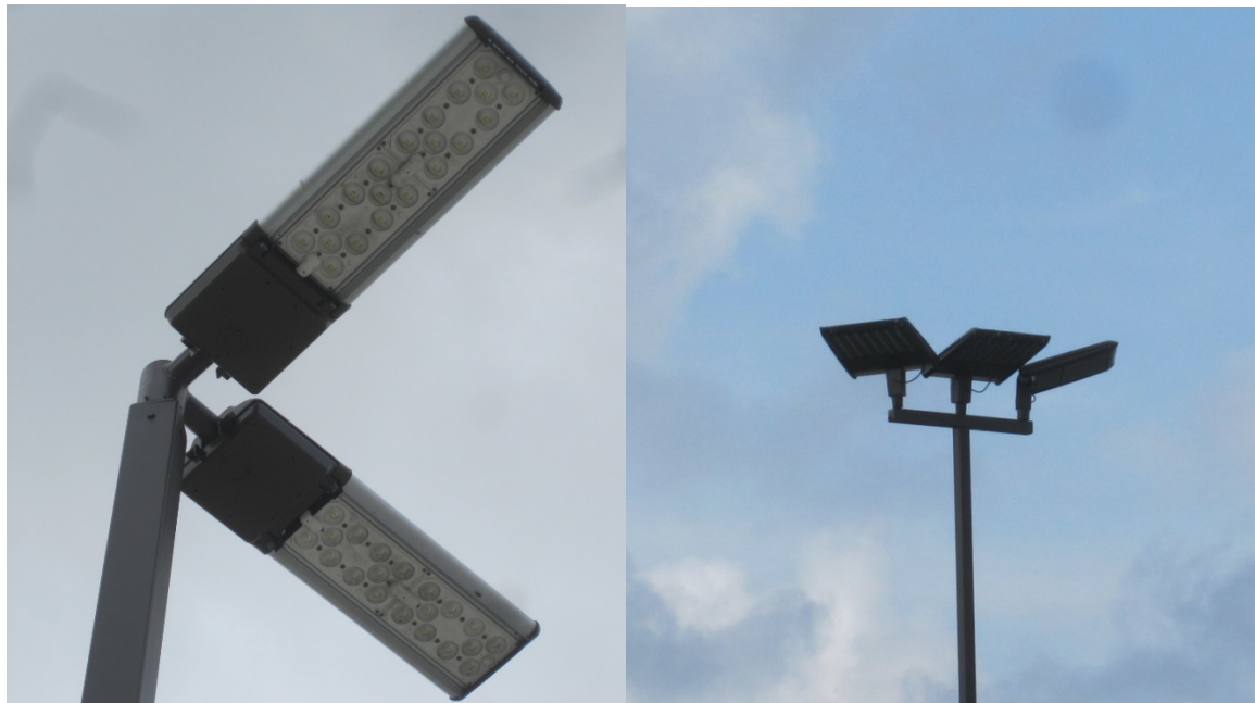
Figure 2-8 LED Area Lighting
