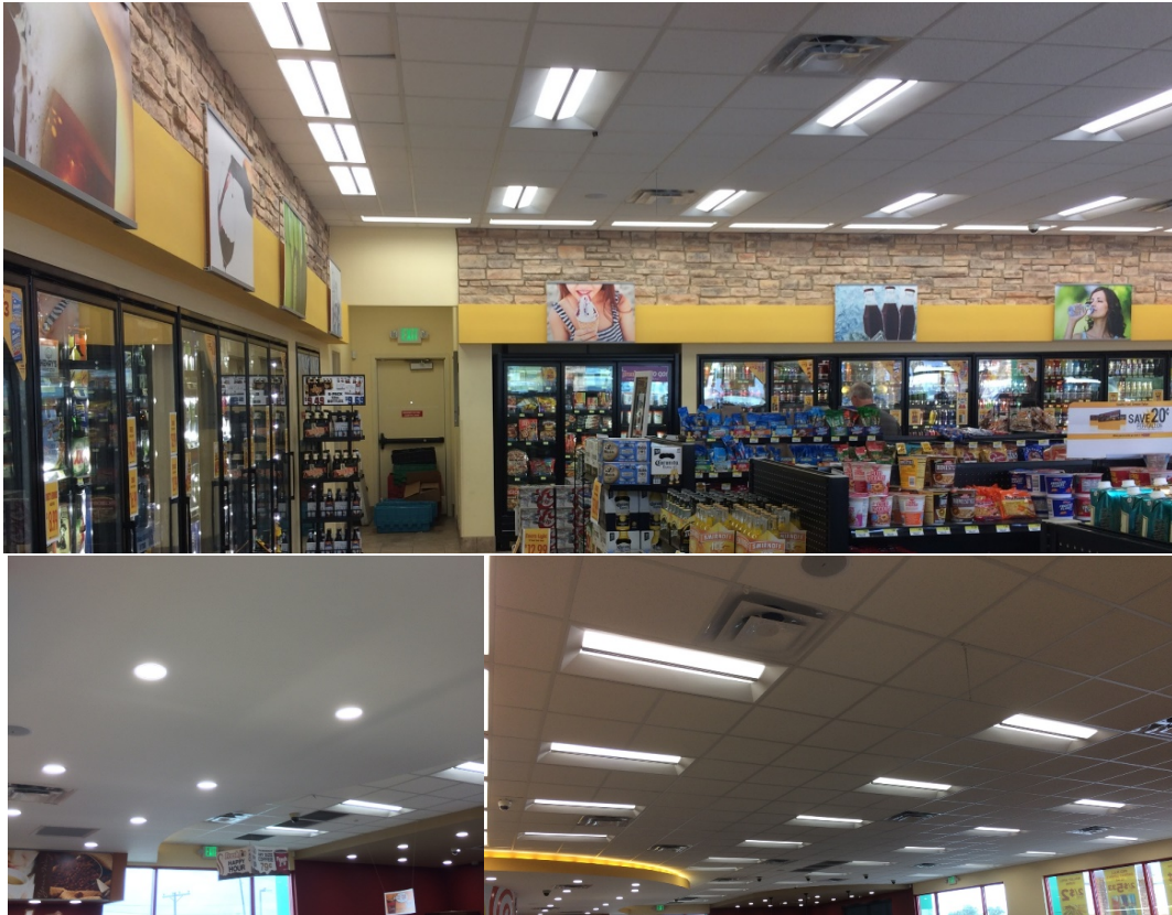
Figure 2-6 LED lighting in the main retail space
