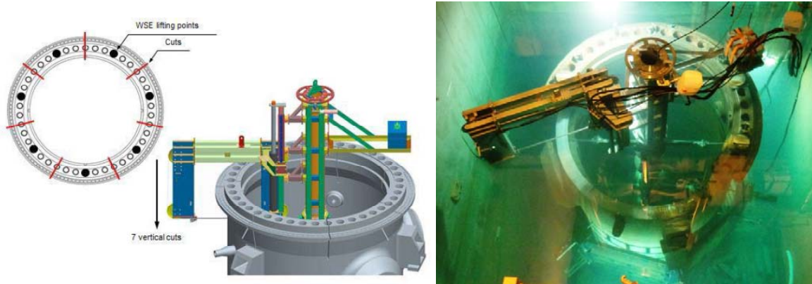
Figure 5-3 Making Vertical Cuts to the Vessel at José Cabrera [27]
