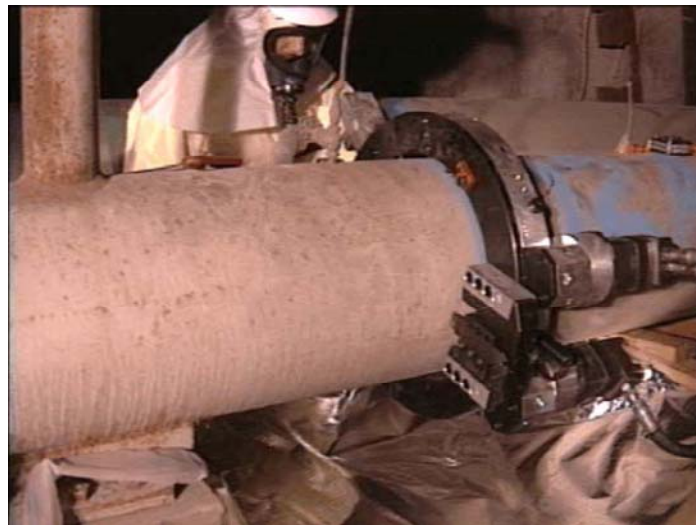
Figure 5-6 High Speed Clamshell Cutter During Demonstrations at Hanford [16]
