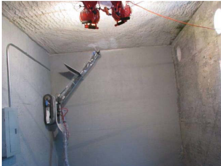
Figure 7-4 CM Climbing Machine Spraying Fixative [16]
