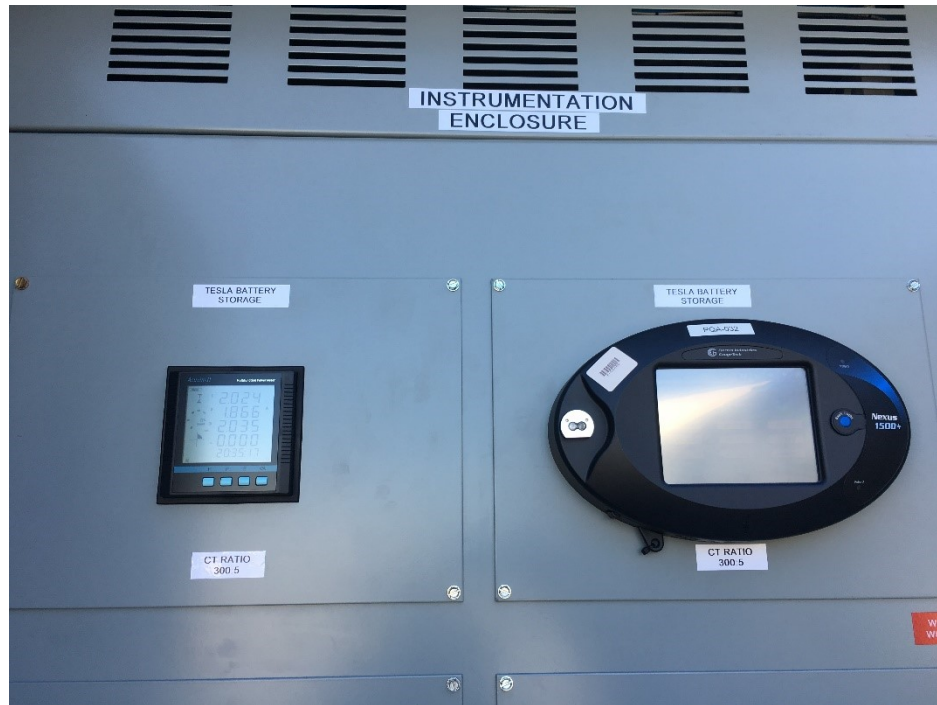
Figure 4-4 Two meters measure the same data points in parallel, specified by Tesla (left) and SCE-installed Nexus 1500 meter (right)
