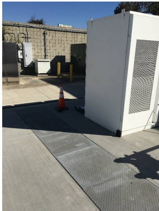
Figure 4-2 Constructed metal plates covering trenches in flexible pad design
