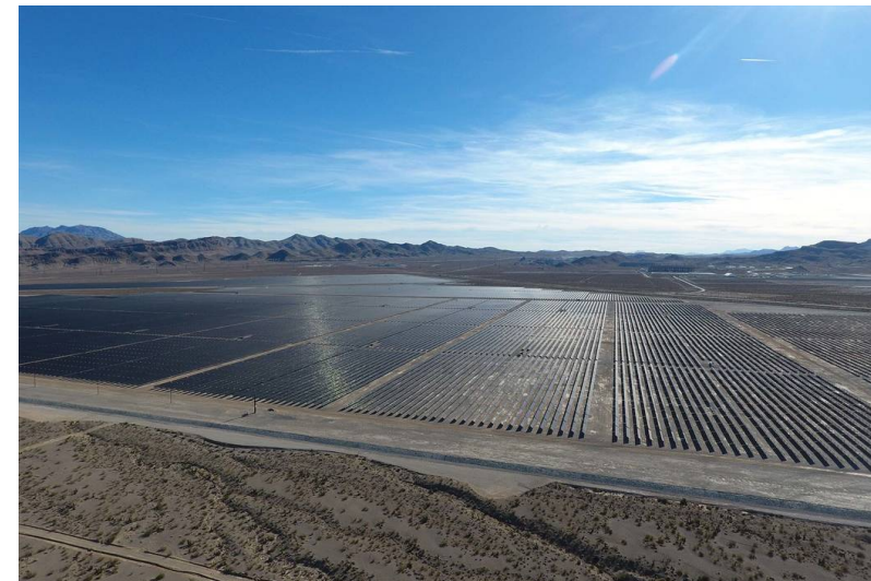
Dry Lake Switch Solar Project, Nevada
