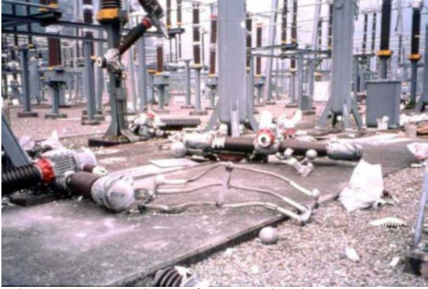
Substation equipment damage from an earthquake.
