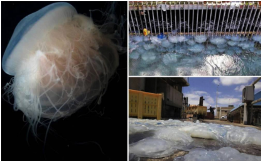
A pink meanie jellyfish feeds on a moon jelly (left, Smithsonian 2013). Hundreds of jellyfish block the trash racks (top right) and cover the floor (lower right) at the Orot Rabin Power Station in Hadera, Israel ( www.dailymail.co.uk ).
