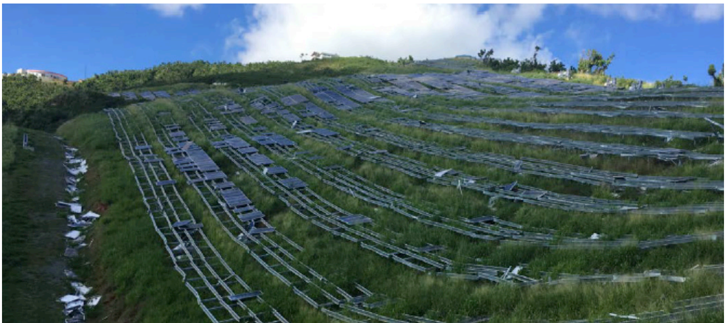
Figure 12 - Hurricanes and other natural disasters are a significant current source of EOL modules. (Photo Credit: Eliza Hotchkiss, NREL)
