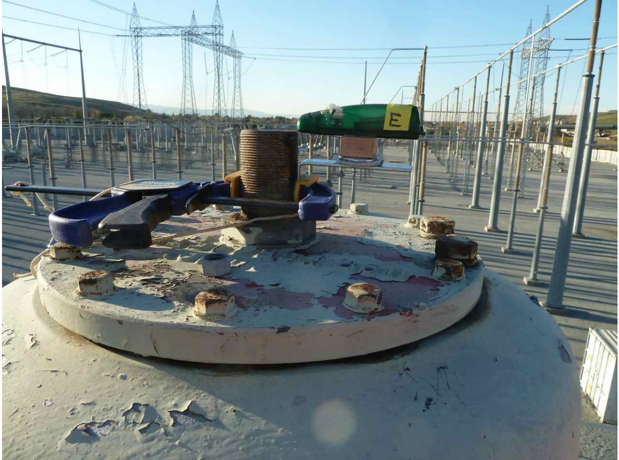
Figure 4-4 Accelerometer attached to 500 kV transformer bushing that is being replaced
