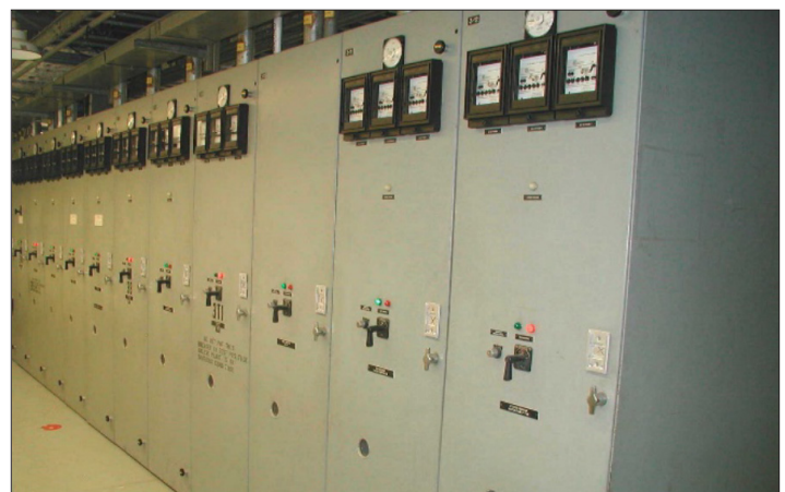
Figure 2 – Medium-voltage switchgear
