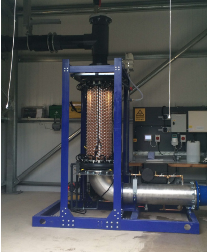
Figure 1. 250 m 3 per hour (~1100 gallons per min) UV-C LED Water Disinfection System Courtesy of Typhon Water Treatment Systems Ltd.
