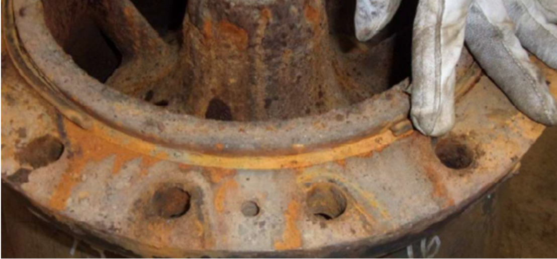
Figure J-7 Failed O-ring caused by bolting failures
