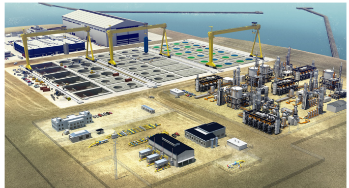
Figure 9. Perspective highlighting the integration of on-site fabrication, assembly, deployment, hydrogen production, and product delivery in a single hydrogen gigafactory. On-site equipment assembly and modular civil works fabrication appear in upper left-hand corner. As nuclear heat source/reactor units and other systems are completed, they are moved via cranes into position in the reactor farm (center) for below-grade installation of heat sources and their companion heat exchanger modules (blue and green hatches) and to the hydrogen production yard (center right). Hydrogen is injected at pressure into the existing natural gas network via underground piping that connects from the hydrogen production facility to compressor stations (black-roofed structures lower center). Graphic courtesy of LucidCatalyst; used with permission.
