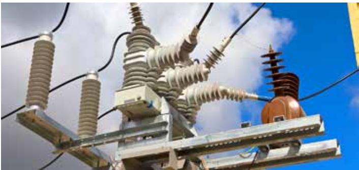
Figure 1 – Some modern protection devices have advanced features to reduce damage to distribution assets, minimize energy into a fault during reclose attempts, and save fuses to reduce the work of field crews.
