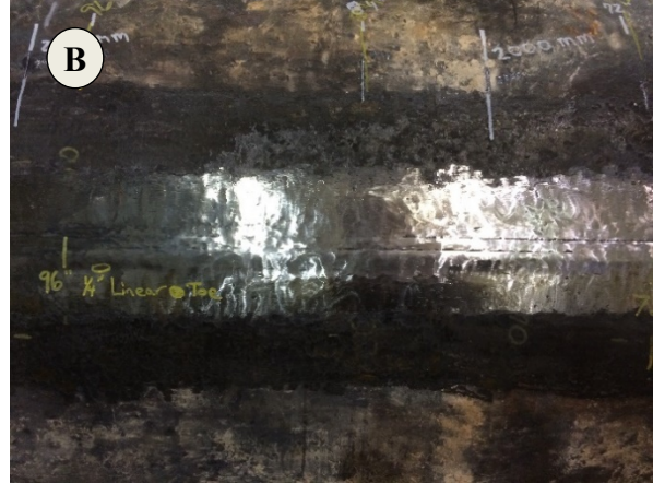
Good manual grinding/final sanding preparation; MT examination detected short weld toe indications
