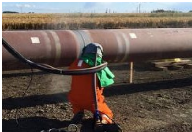
Figure 2-6 Example of dry abrasive blasting (sandblasting)
