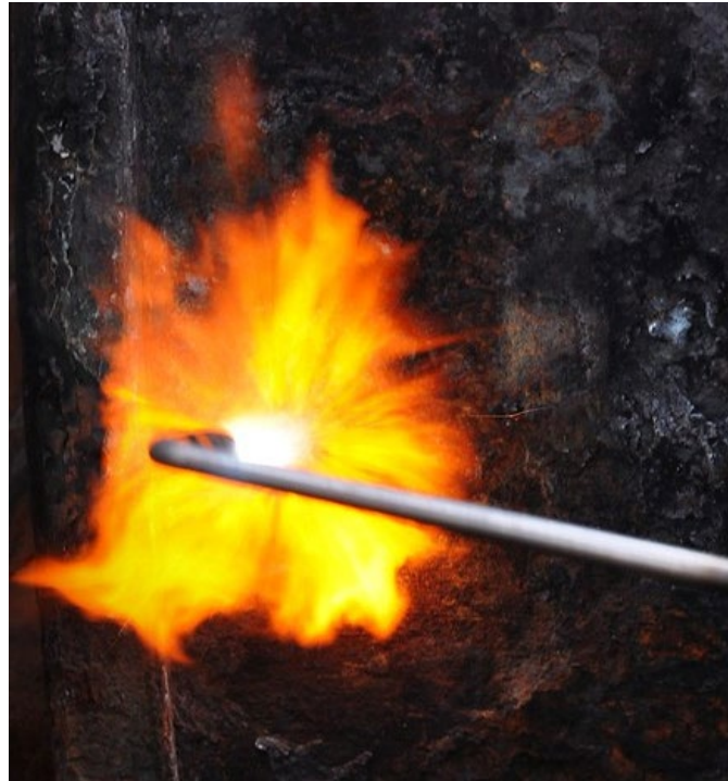
Figure 2-27 Example of thermal descaling using an oxy-acetylene rosebud torch
