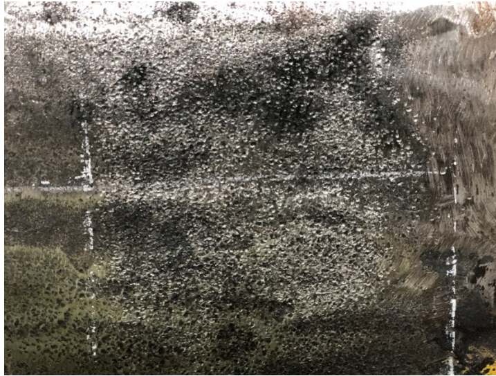
Figure 2-26 Example surface peened by excessive pressure during needle descaler operation. This surface will require additional finishing/smoothing with 40-to-120-grit sanding disks.
