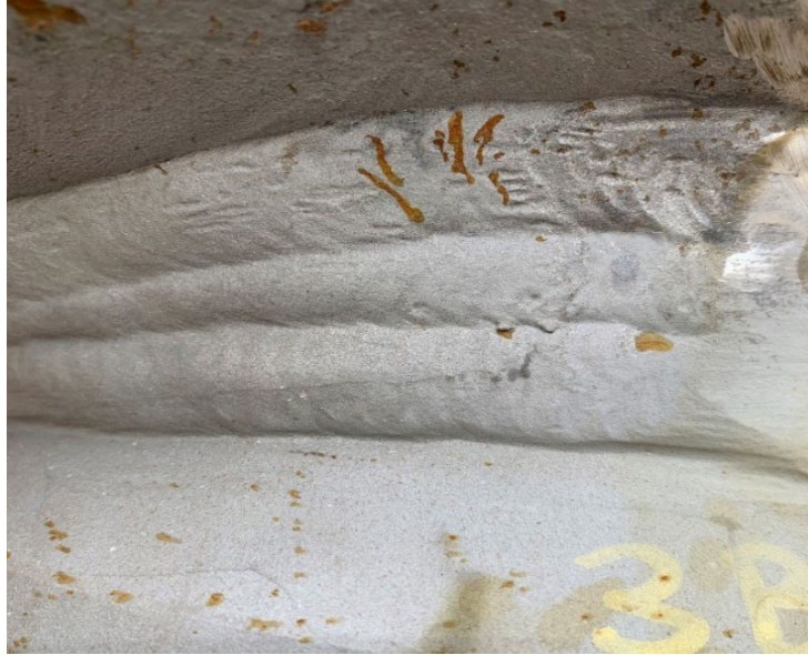
Figure 2-9 Example of wet abrasive blasting surface after cleaning
