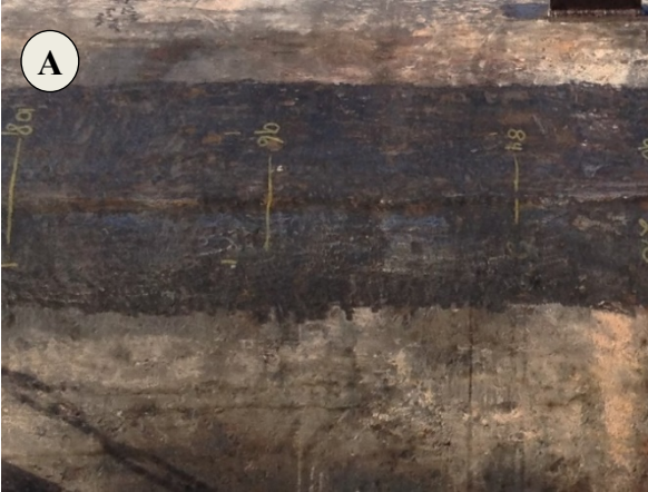
Bad manual grinding preparation; areas of scale left, and MT examination detected no indications
