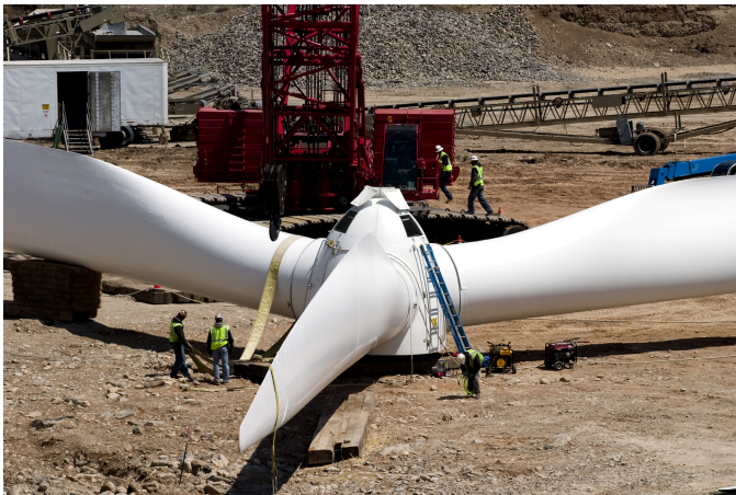
Figure 4. Wind turbine blades being removed.
