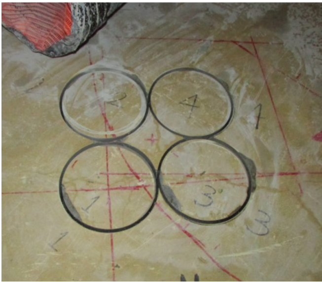
Figure 3-2. Top surface of the concrete after wet coring (left) and bottom of the cavity a few centimeters away from the plate (right) (Used with permission from Energy Harbor.)
