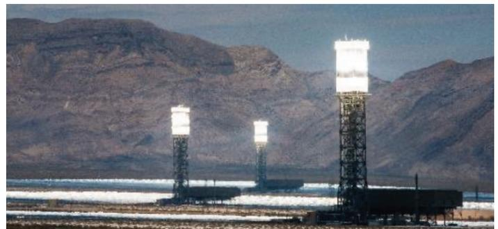
Figure 13. The proposed 50-MW<sub>e</sub> modular design would shorten project construction time while allowing for larger, multi-unit facilities if desired. Photo: Ivanpah Solar Electric Generating Station, USA (Courtesy of NREL)
