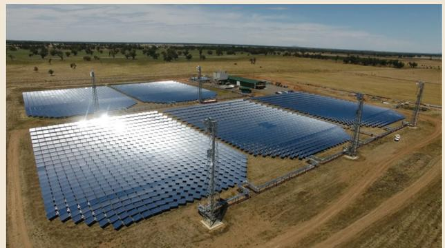
Figure 9. Vast Solar's 5-MW<sub>th</sub> (1.1 MW<sub>e</sub>) Jemalong pilot facility (Courtesy of Vast Solar)
