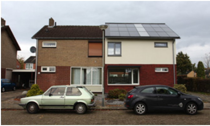
Figure 6: Net-zero energy retrofit completed using the Energiesprong approach
