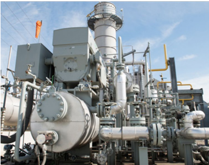
Figure 8. Site photo of Southern California Edison’s Center Hybrid Enhanced Gas Turbine (left) and interior view of the integrated gas turbine and battery storage system controls compartment.
