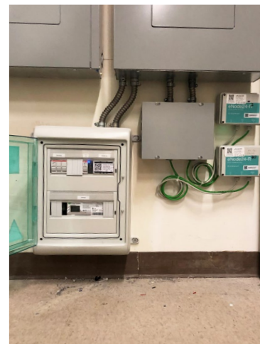
Networked metering, sensing, and communications hardware deployed at EPRI's headquarters provided the data required for optimizing HVAC control to reduce energy consumption without impacting thermostat settings.
