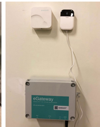
Networked metering, sensing, and communications hardware deployed at EPRI's headquarters provided the data required for optimizing HVAC control to reduce energy consumption without impacting thermostat settings.
