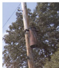
Corroded Transformers
