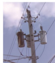
Corroded Transformers
