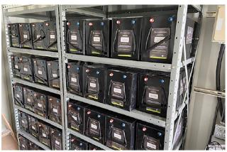
Like other stationary storage battery platforms, UEP's technology offers the advantages of modularity—but ZnMnO<sub>2</sub> batteries also are based on materials that are globally abundant and not subject to thermal runaway.
