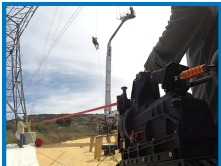
Figure 18: Battery-powered ascender devices for direct access to conductors
