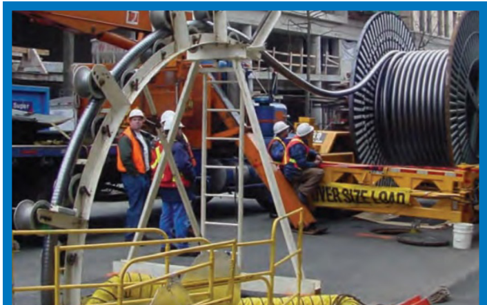
Figure 12: Installation of underground cable in an urban area
