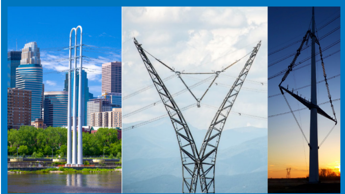
Figure 7: Examples of aesthetic transmission lines [Images courtesy of Nigel Young/Foster + Partners and RTE]
