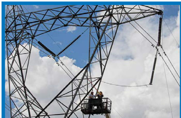
Figure 17: Installing a Portable Protective Arrester [7]
