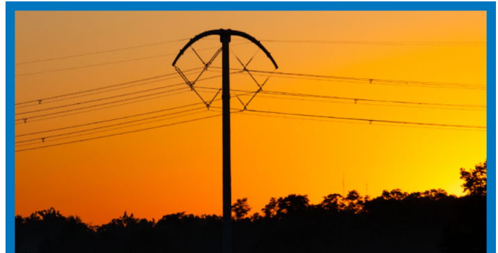
Figure 23: Hybrid implementation of BOLD, including 138kV and 345kV circuits [Courtesy of BOLD Transmission, LLC]
