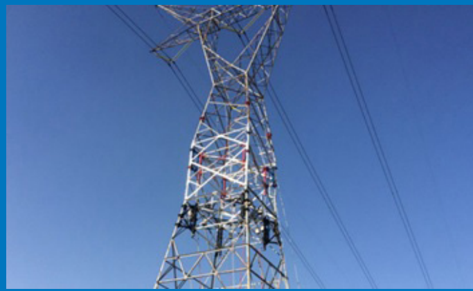
Figure 8. Raising of lattice tower for clearance enhancement [Courtesy of Ampjack]
