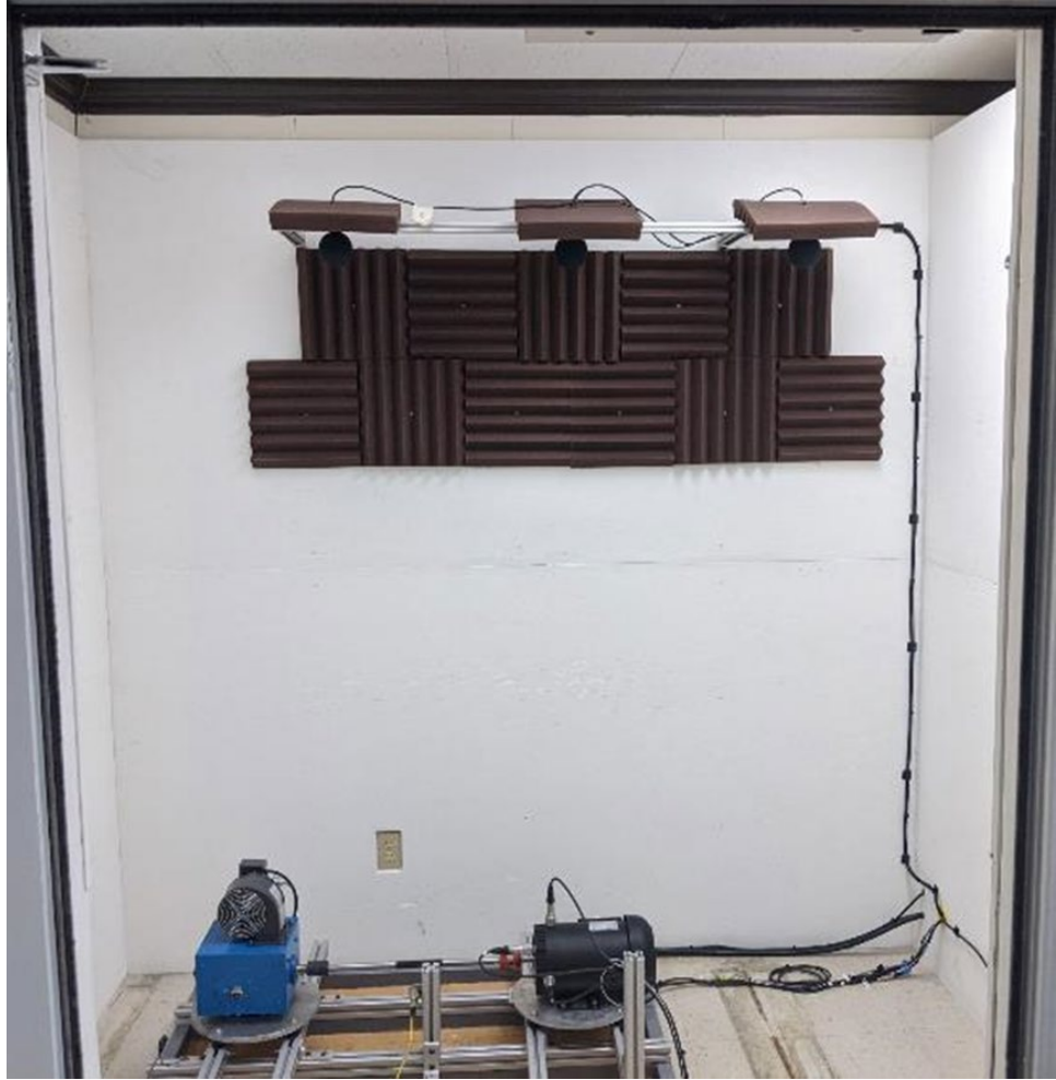
Figure 3-2 Acoustic array installed in the test chamber
