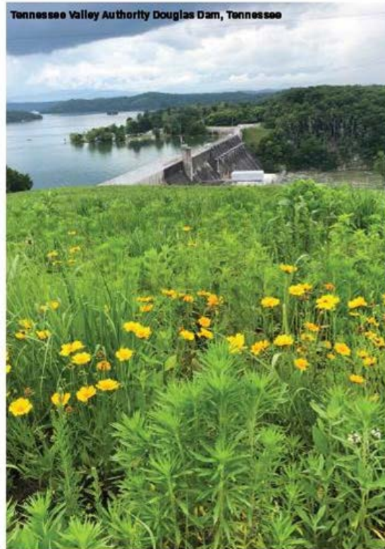
Figure 3-4 Pollinator habitat in the upland area of a hydro generating site Credit: EPRI 2021 Pollinator Power Party Calendar (3002020257)
