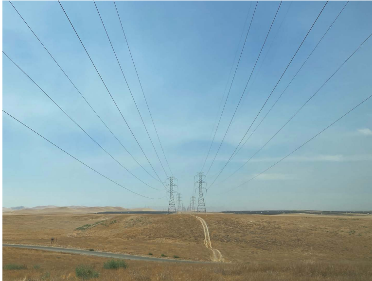
Figure 3-1 Transmission corridor in California with ground mounted solar in the distance Credit: S. Frischie, The Xerces Society
