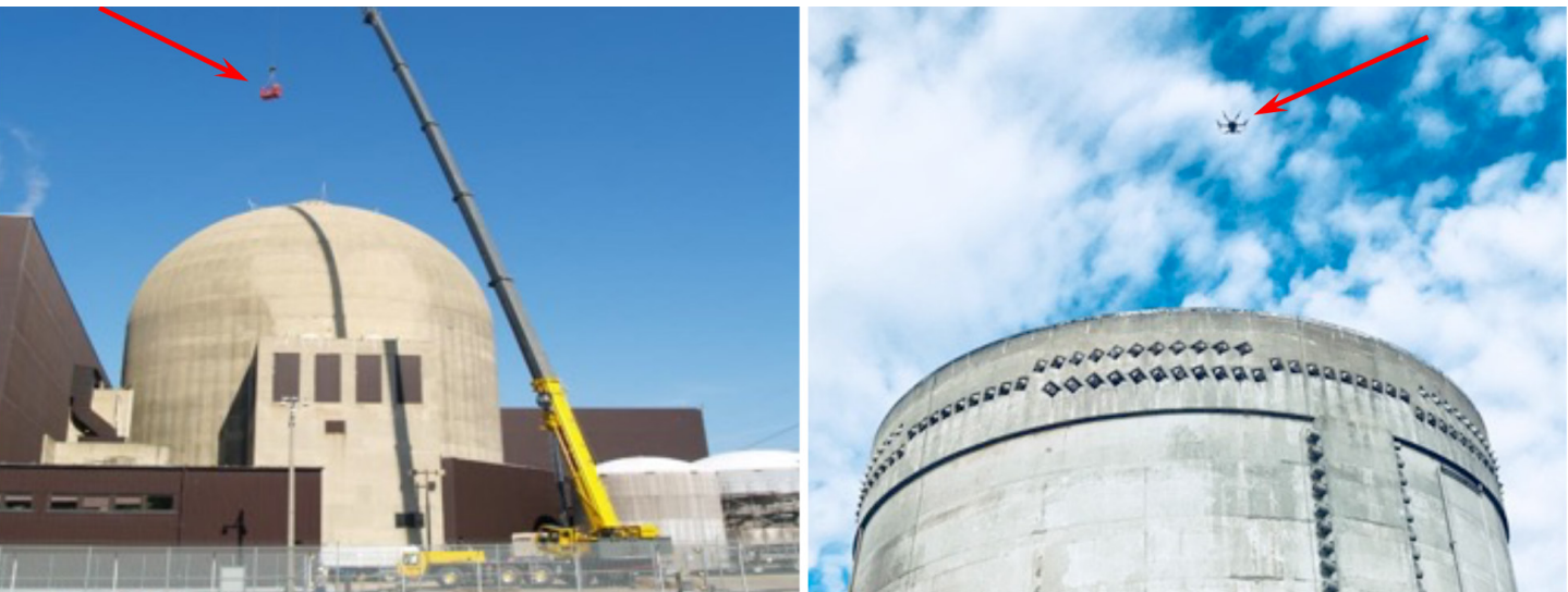
Figure 1 – Manual (Left) and drone (right) visual inspection of a containment structure
