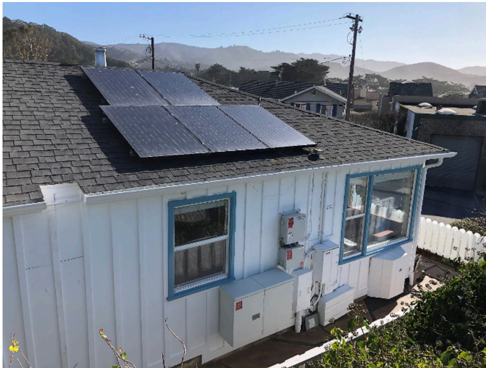
Figure 2. Typical Residential Customer-Sited BESS and Solar Installation in Pacifica, California Source: EPRI
