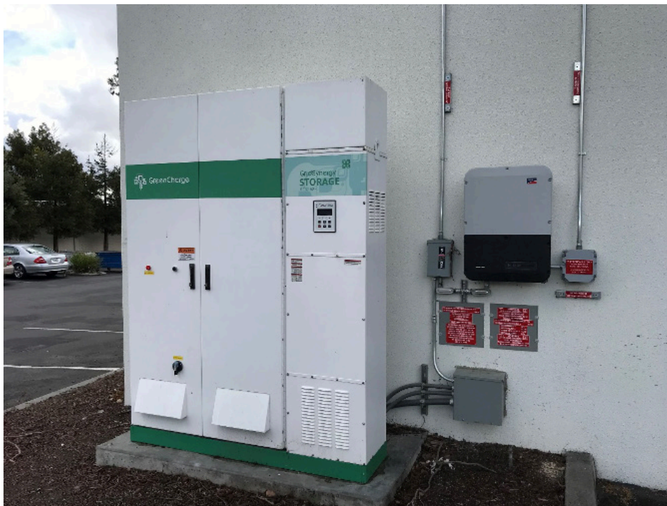
Figure 3. Commercial Customer-Sited BESS Installation in San Jose, California Source: EPRI
