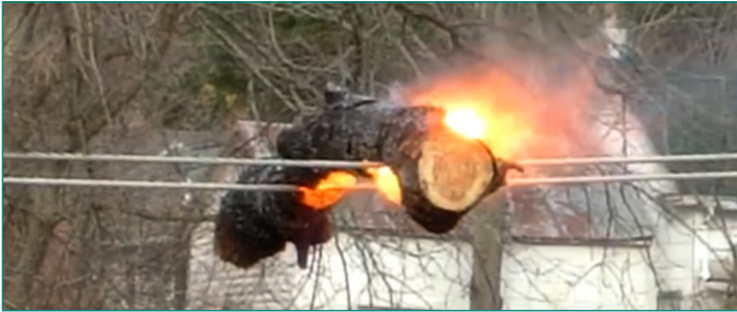
Figure 3. Tree-limb phase to phase
