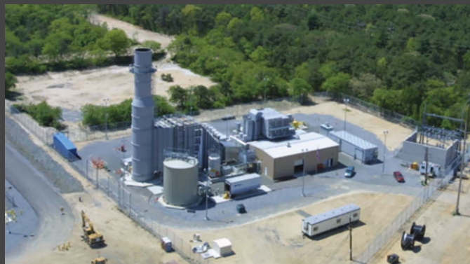
Figure 1. Aerial view of Brentwood Facility.
