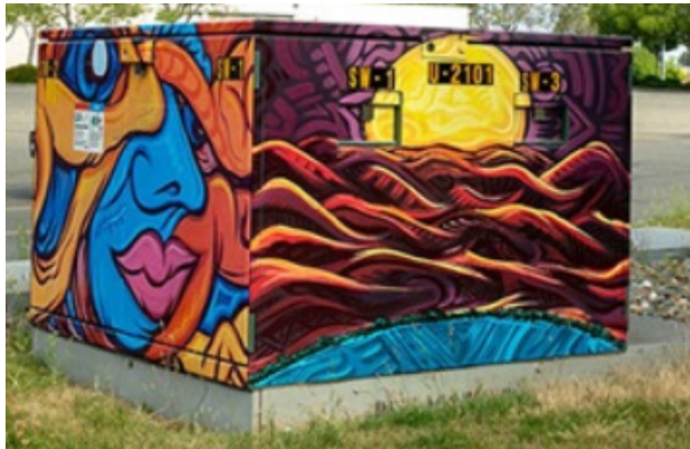
Aesthetic wrap applied to padmount switchgear in the field
