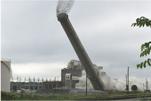
Stack at a fossil-fueled plant being felled
