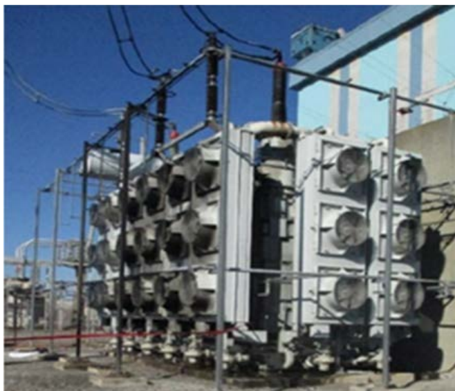
Figure 6. GSU Transformer External View: Catastrophic Failure of HV Bushing Center Phase
