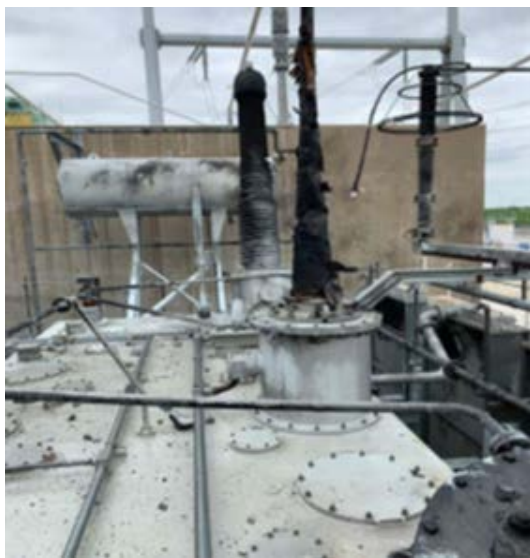
Figure 14. Illustration of A-Phase HV Bushing and Mounting in a Turret with a Surge Arrestor
