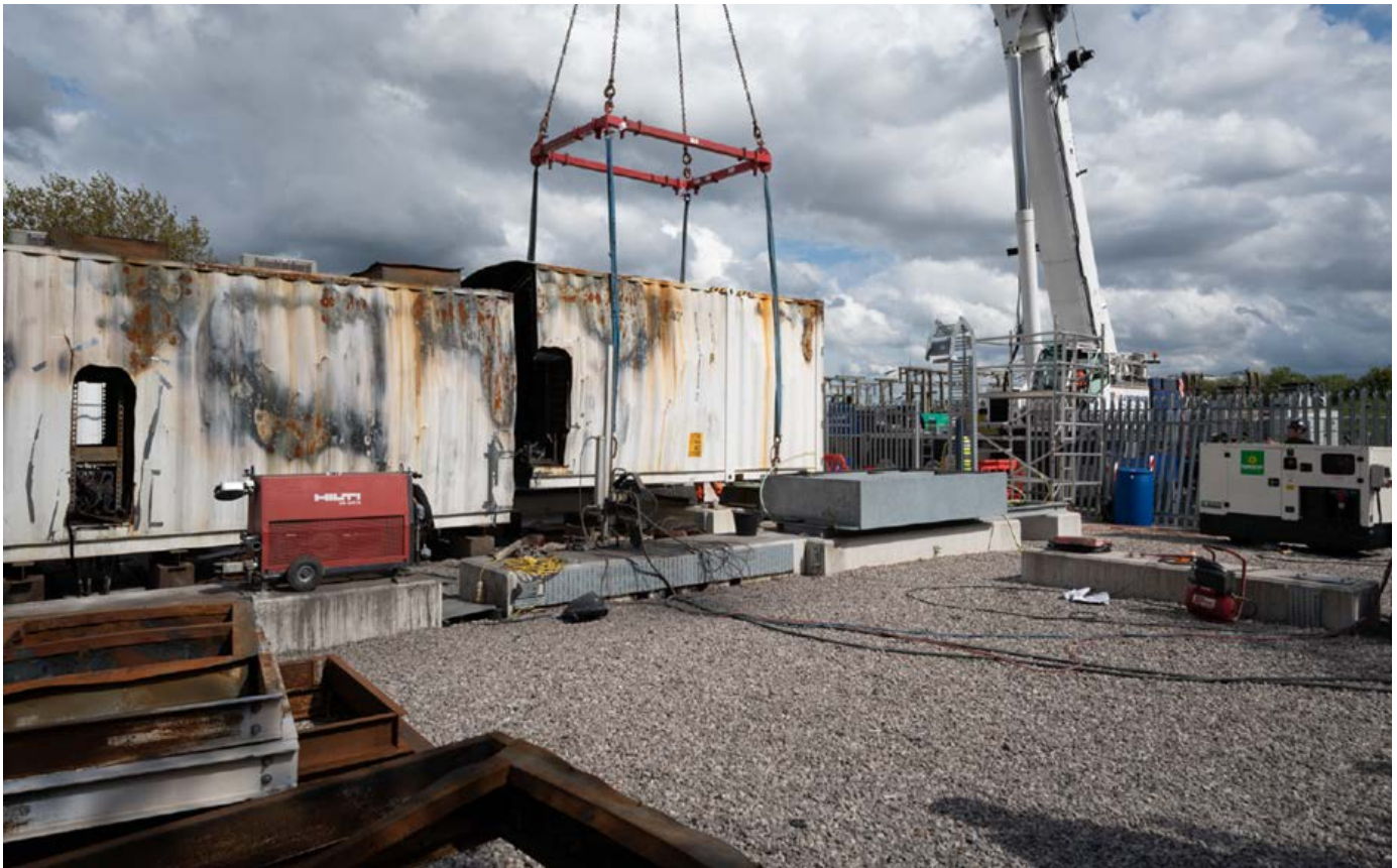
Figure 5 View of Container 1, Section 1 being removed (source: SAFE Laboratories and Engineering Corp.)
