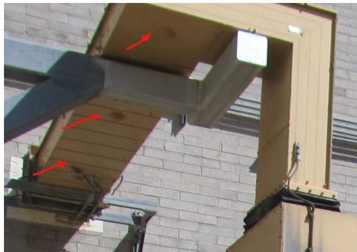
Figure 11-2 Attendee provided photo of bus duct with breathers
