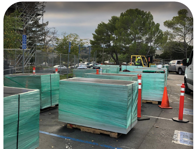
Figure 1. Plastic-wrapped pallets of PV modules awaiting transport to a reuse and recycling center during decommissioning of 187 kW DC rooftop PV system at EPRI's Palo Alto, California headquarters buildings, 2019
